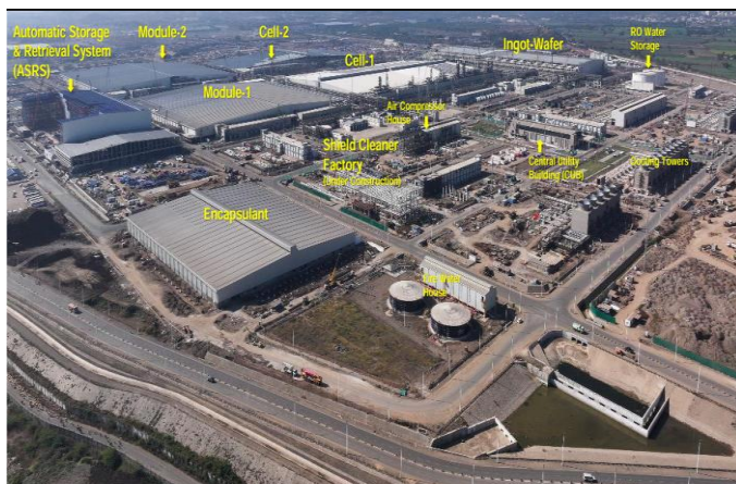
Fig 17 – Construction site overview
